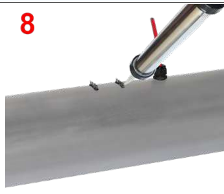
8: Inject sealant around the legs
